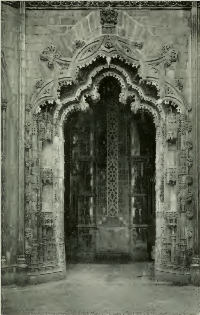
DOORWAY OF THE UNFINISHED CHAPELS, BATALHA
